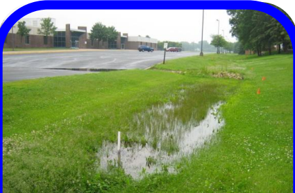
An existing 1,320 foot long drainage swale with poorly draining soils provided little water quality treatment .
