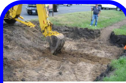
1,820 square feet of infiltration area was created by replacing 150 cubic yards of poorly drained soil with a 70% sand and 30% compost soil mixture.
