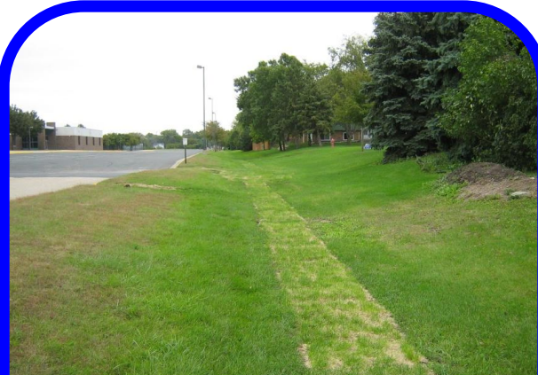
Mowed infiltration areas are integral to the surrounding landscaping. No special maintenance is required.
