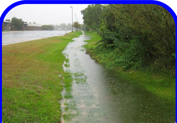
Amended soil turf Infiltration area during a rain event. Surface ponding completely infiltrated within six hours following the rain event.
